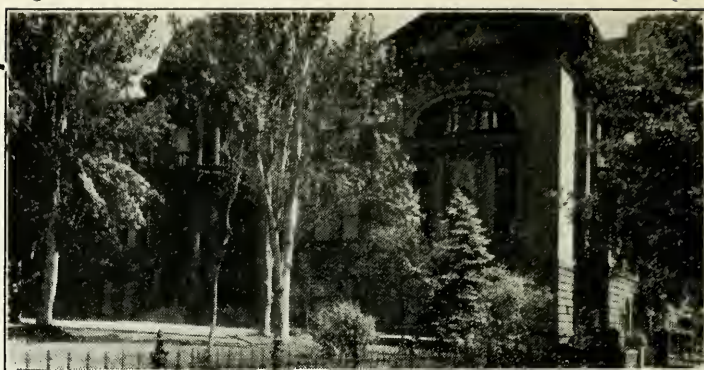
Brigham Young Memorial Building (Home of Y. M. M. I. A. General Offices in Salt Lake City)
